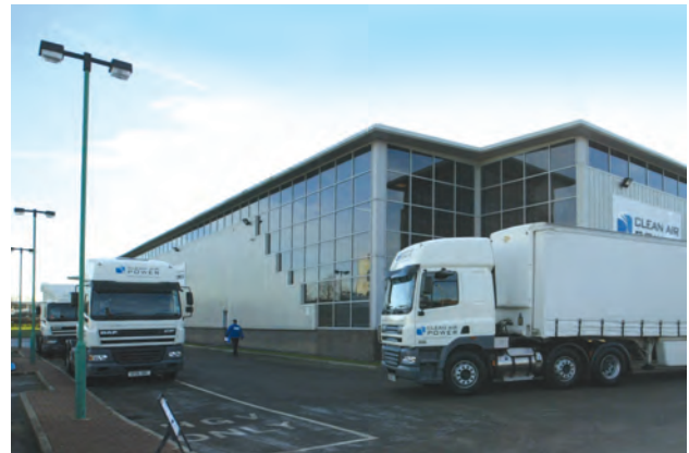
UK Production, R&D and Administration centre, Leyland, Lancashire
