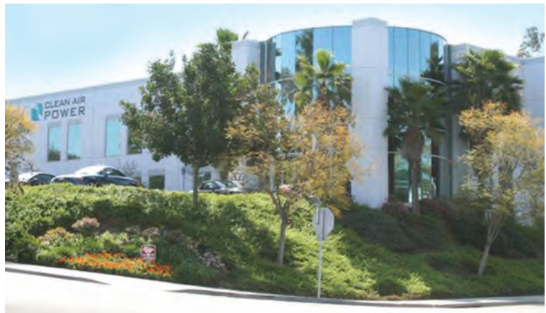
Manufacturing and Research & Development Operations, San Diego, California.
